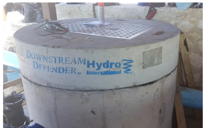
Sediment Separator Installation
